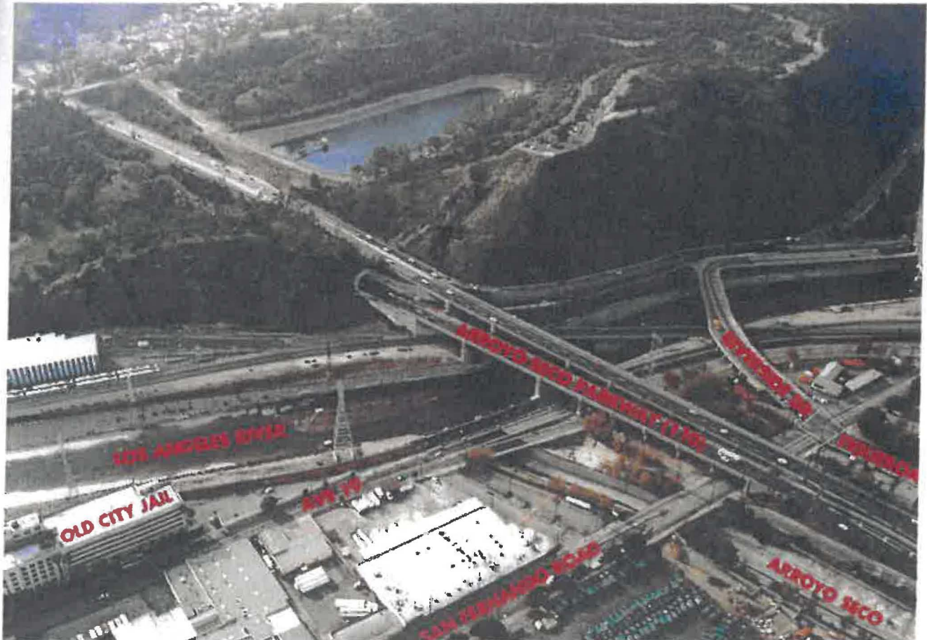
THE MAINTENANCE SHED AT MIDWAY YARD IS SEEN AT THE LEFT EDGE OF THE PHOTO.
